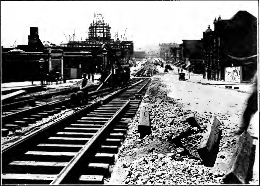
CONSTRUCTION OF VAN NESS AVENUE MUNICIPAL RAILWAY
